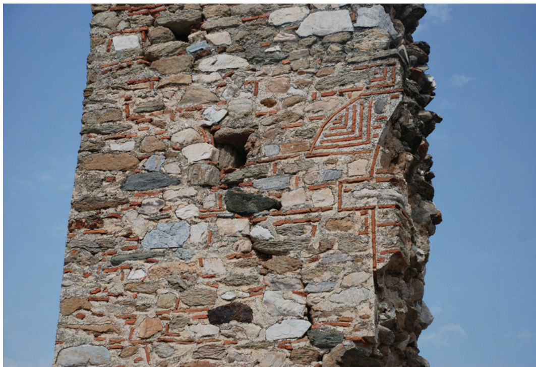
Plate 52. Serbia. Tower of the citadel, masonry detail. (Photo: Flora Karagianni)
